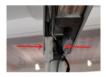
Remove the OP light head by untightening the pinol bolt.
