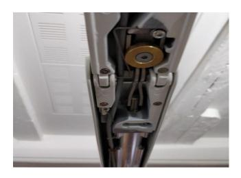
Disconnect the cables from the OP light head.
