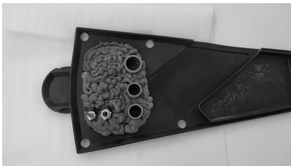
Figure 13 – sealing the floor installations with flame-retardant foam
