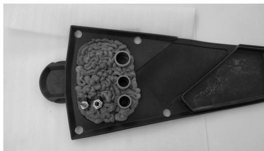
**Figure 12 – Sealing the floor installations with flame-retardant foam**
