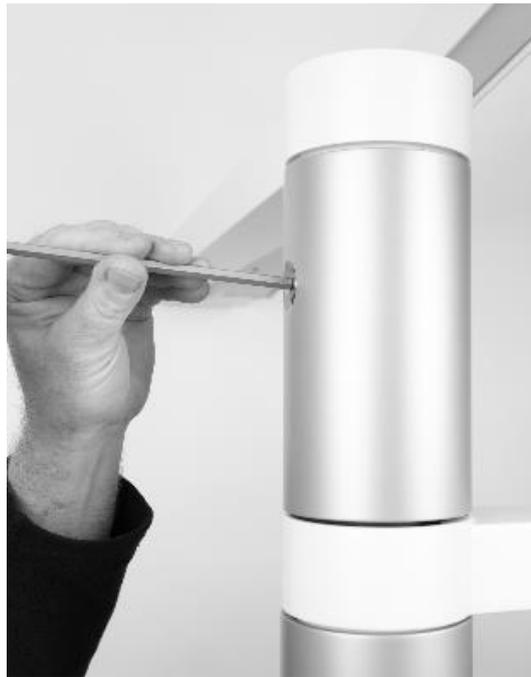
Figure 53 – Fitting the brake
